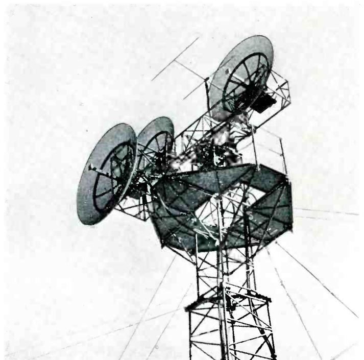
Fig. 4.—Second antenna installed on tower at Catalina for space diversity transmission with Frazier Mountain.
